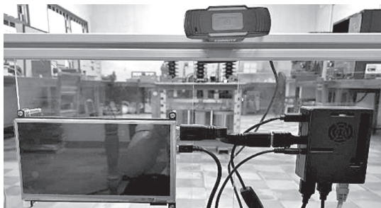
Figure 6. Installation of object recognition and handling equipment.
